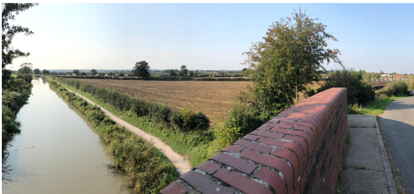
Photograph from canal bridge facing westwards - September 2020
